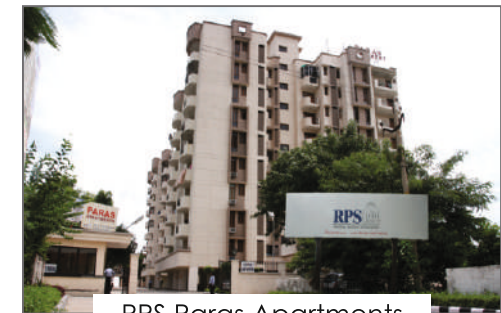
RPS Paras Apartments
